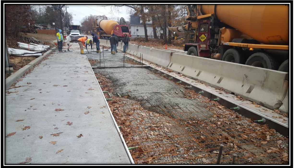
Figure: 2 – Installation of concrete surface course in the northbound travel lane in the vicinity of the intersection with Cloverdale Avenue
