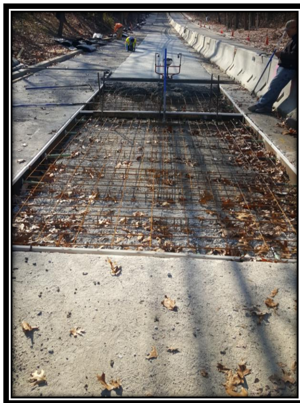
Figure: 1 – Wire mesh and dowel reinforcement of concrete surface course installation in the northbound travel lane in the vicinity of the intersection with Cloverdale Avenue
