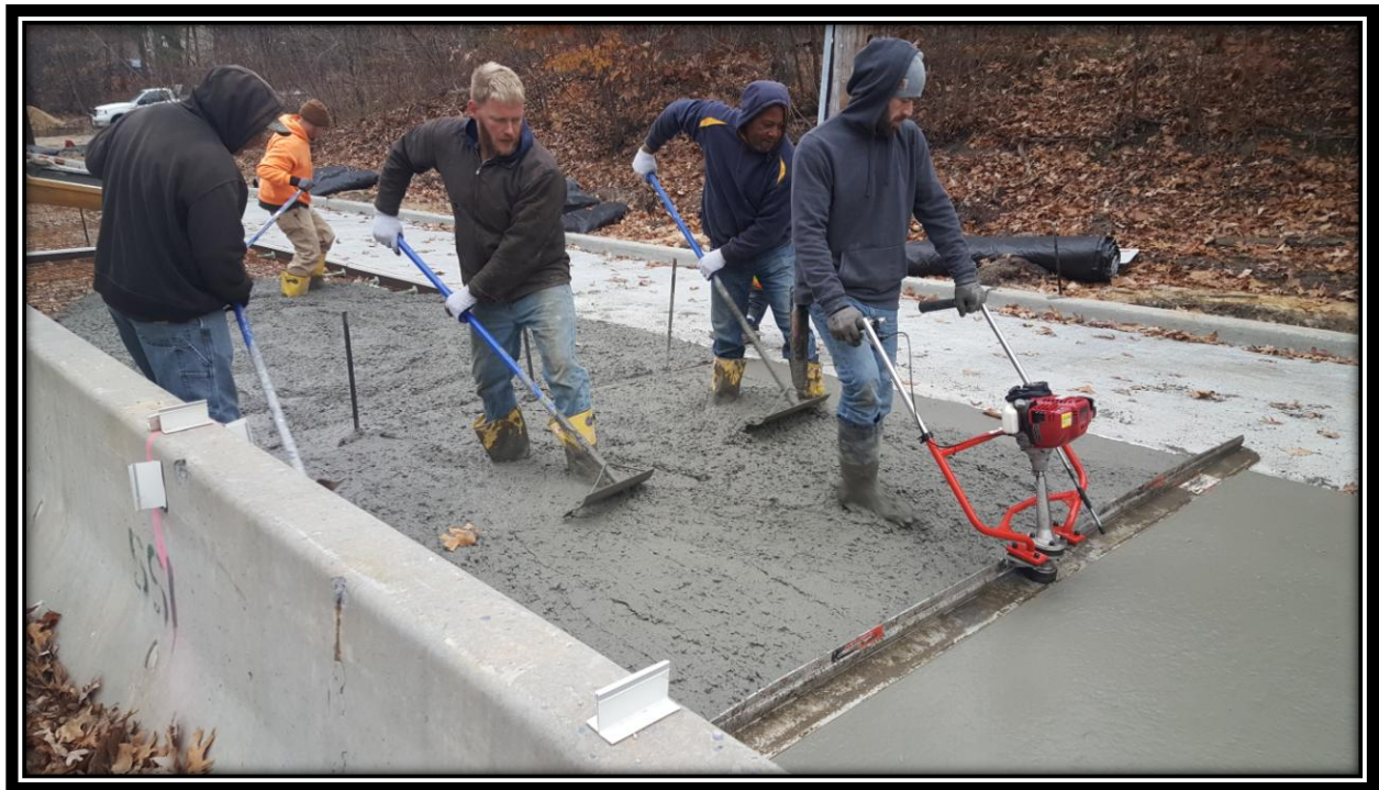
Figure: 3 – Finishing of concrete surface course in the northbound travel lane in the vicinity of the intersection with Cloverdale Avenue
