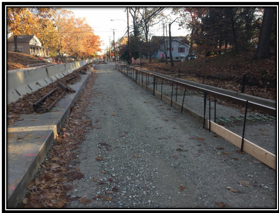
Figure: 1 – Installation of dowels in preparation of concrete surface course installation in the northbound shoulder in the vicinity of the intersection with Cloverdale Avenue
