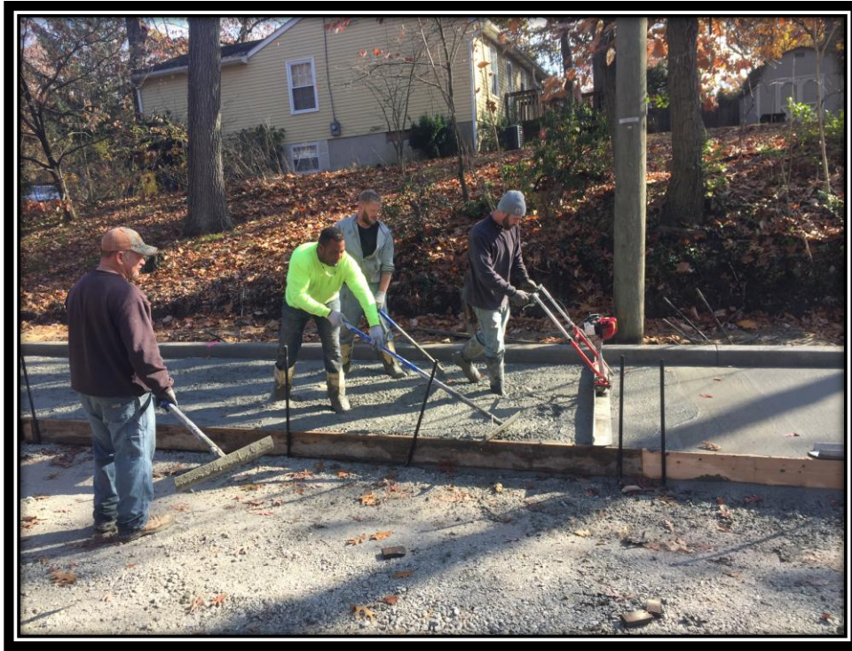
Figure: 2 – Installation of concrete surface course in the northbound shoulder in the vicinity of the intersection with Cloverdale Avenue
