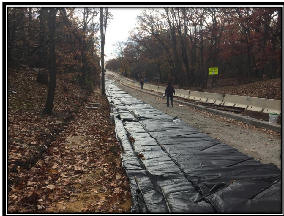
Figure: 3 – Installation of thermo blankets to protect the newly installed concrete surface course in the northbound shoulder in the vicinity of the intersection with Cloverdale Avenue
