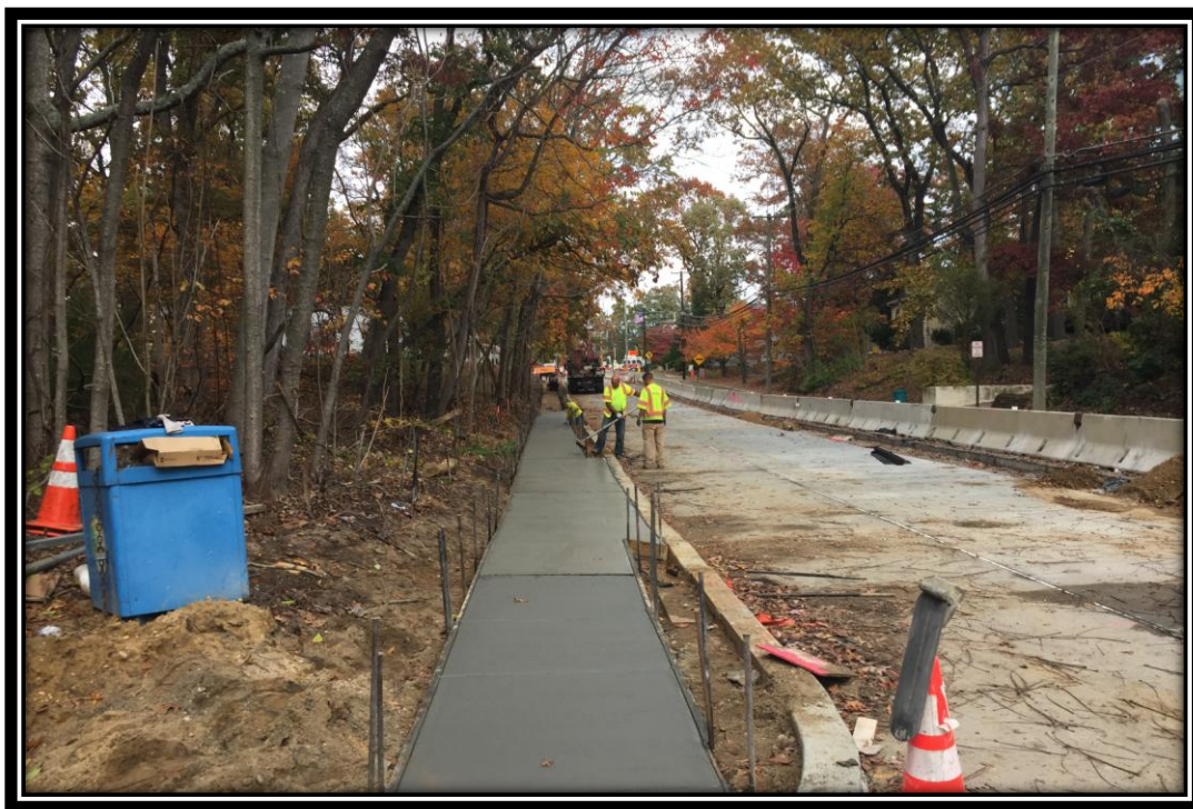
Figure: 1 – Installation of concrete sidewalk and driveway apron along the southbound lane in the vicinity of the intersection with Cloverdale Avenue
