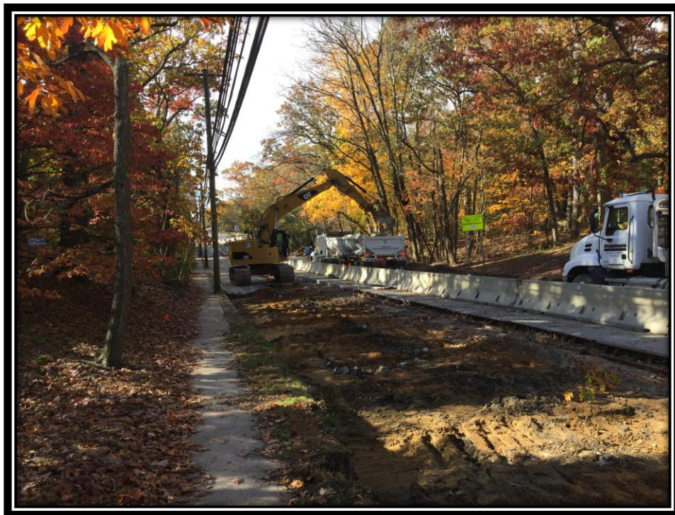
Figure: 3 – Removal of existing concrete roadway in the northbound lane in the vicinity of the intersection with Cloverdale Avenue
