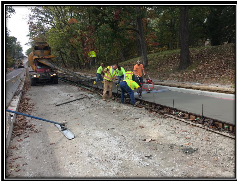
Figure: 3 – Installation of 8 inch thick concrete surface course in the southbound lane in the vicinity of the intersection with Cloverdale Avenue
