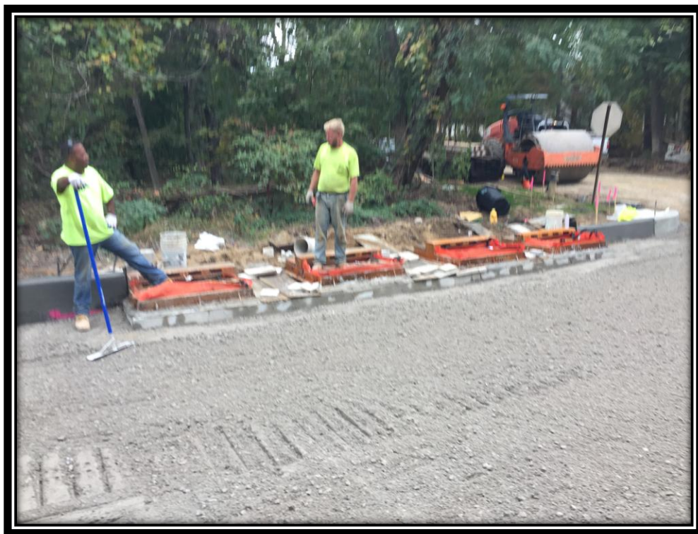
Figure: 1 – Installation of 8" thick dense graded aggregate base course in the southbound lane in the vicinity of the intersection with Cloverdale Avenue
