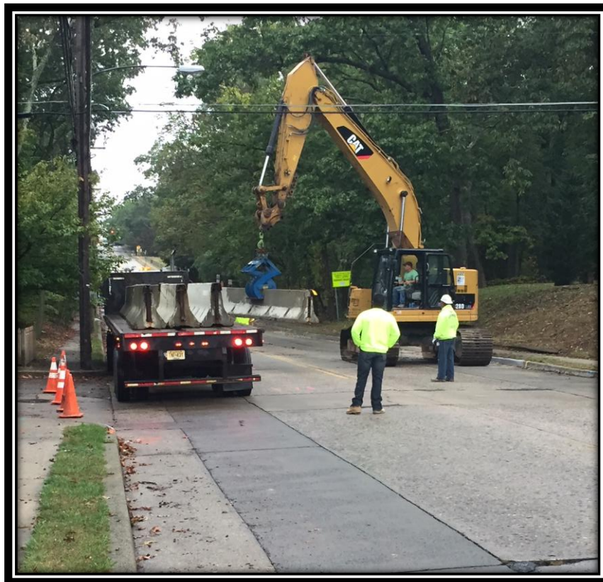
Figure: 1 – Installation of traffic control measures in the vicinity of the intersection with Cloverdale Avenue
