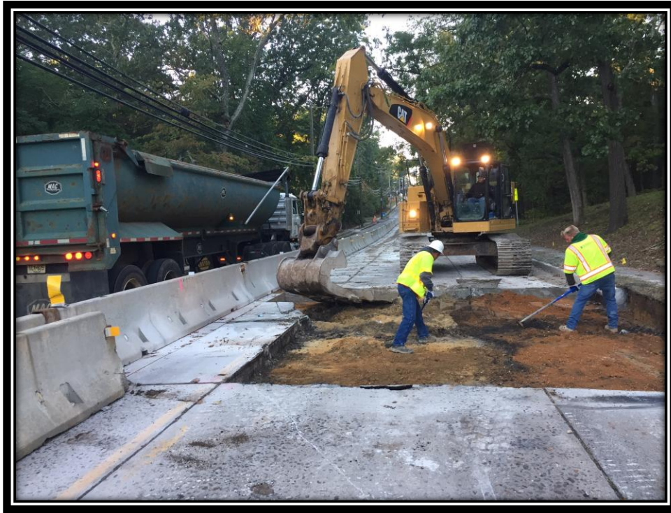
Figure: 2 – Removal of existing concrete surface course in the southbound lane in the vicinity of the intersection with Cloverdale Avenue
