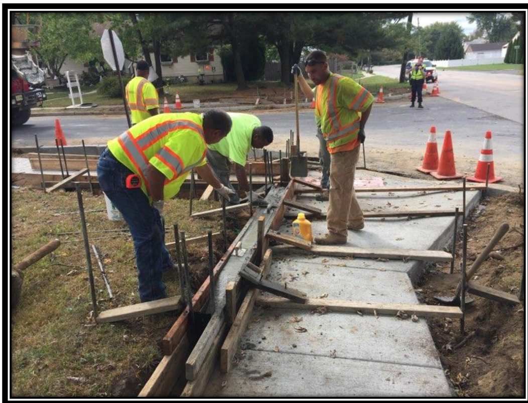
Figure: 1 – Installation of ADA ramp along the eastbound lane at the southwest corner of the intersection with Danbury Drive
