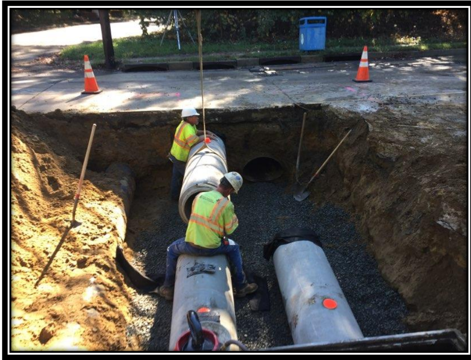
Figure: 2 – Installation of triple 18" RCP storm sewers at the intersection with Cloverdale Avenue
