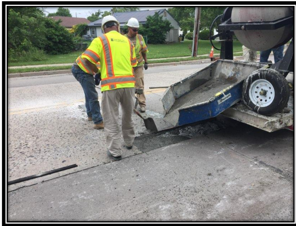
Figure: 3 – Partial depth concrete slab repairs in the northbound lane between Danbury Drive and Shultz Avenue
