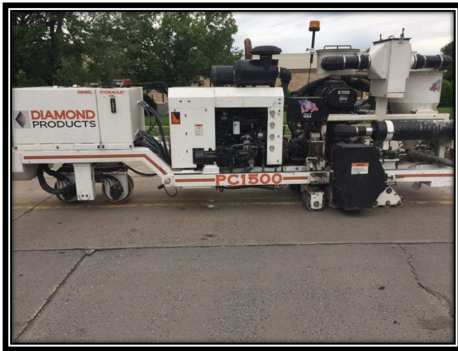
Figure: 2 – Diamond grinding of the concrete surface course in the northbound lane between Erial New Brooklyn Road and Pleasantview Drive
