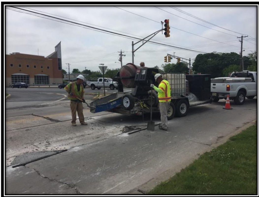
Figure: 1 – Partial depth concrete slab repairs in the southbound lane approaching the intersection with Erial New Brooklyn Road
