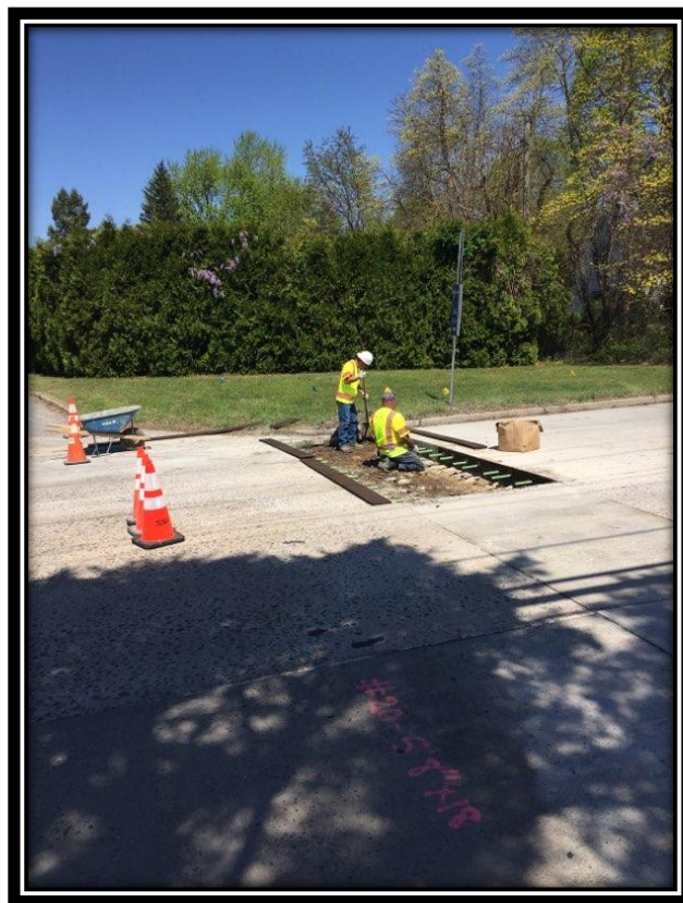
Figure: 1 – Preparation of full depth concrete slab repair along the southbound lane between Bromley Drive and Shultz Avenue
