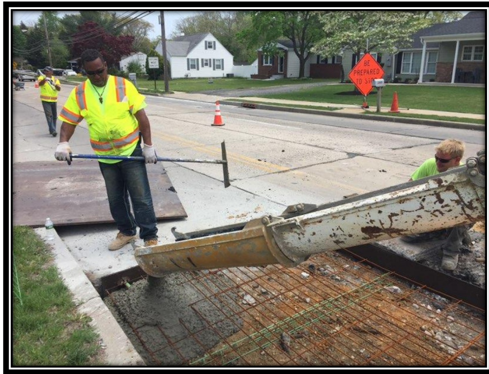
Figure: 2 – Full depth concrete slab repair along the southbound lane between Bromley Drive and Shultz Avenue
