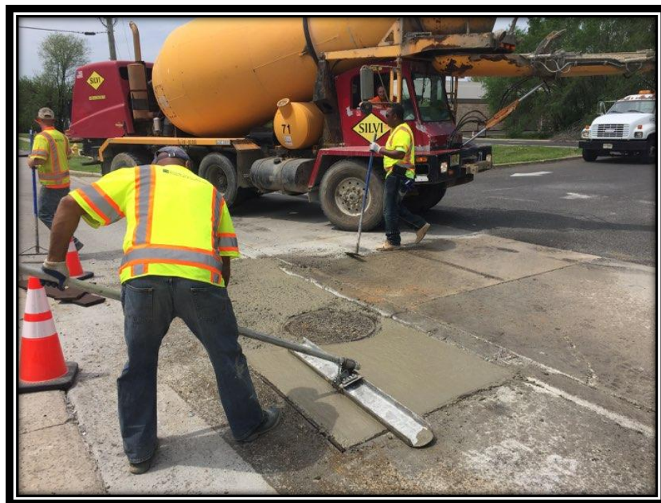
Figure: 3 – Full depth concrete slab repair along the southbound lane at the intersection with Pleasantview Drive
