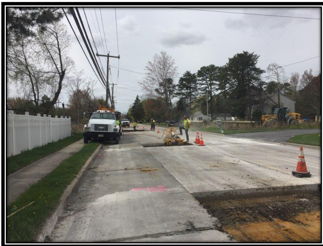
Figure: 1 – Preparation of full depth concrete slab repair along the northbound lane between Shultz Avenue and Bromley Drive
