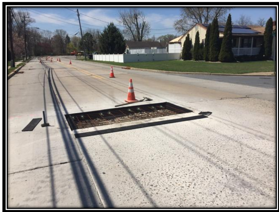
Figure: 3 – Full depth concrete slab repair along the northbound lane between Pleasantview Drive and Lee Lane
