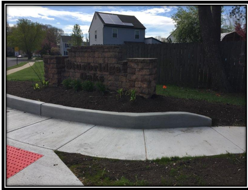
Figure: 2 – Topsoil and seed restoration at the newly installed ADA ramp at the intersection with Bromley Drive
