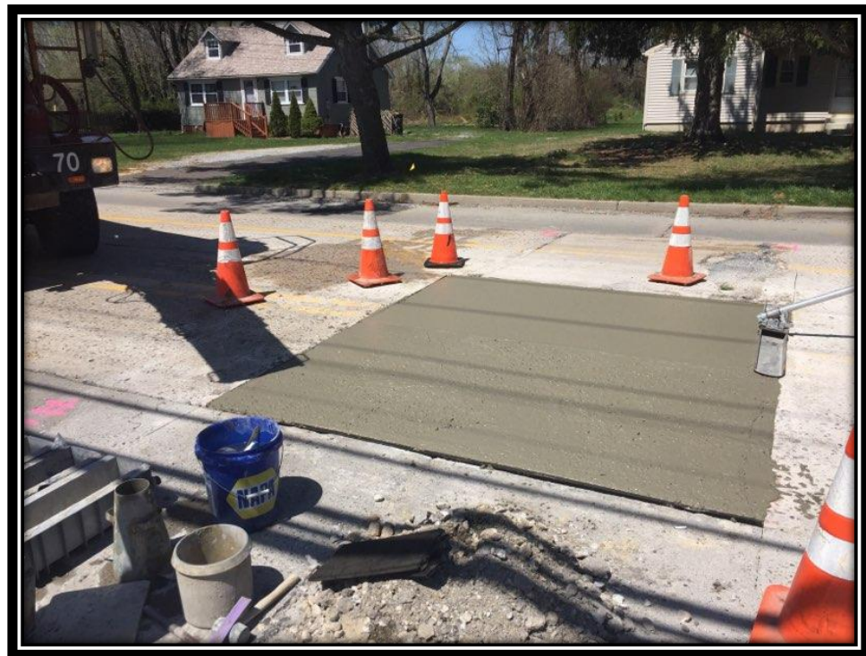
Figure: 3 – Full depth concrete slab repair along the northbound lane between Erial - New Brooklyn Road and Pleasantview Drive
