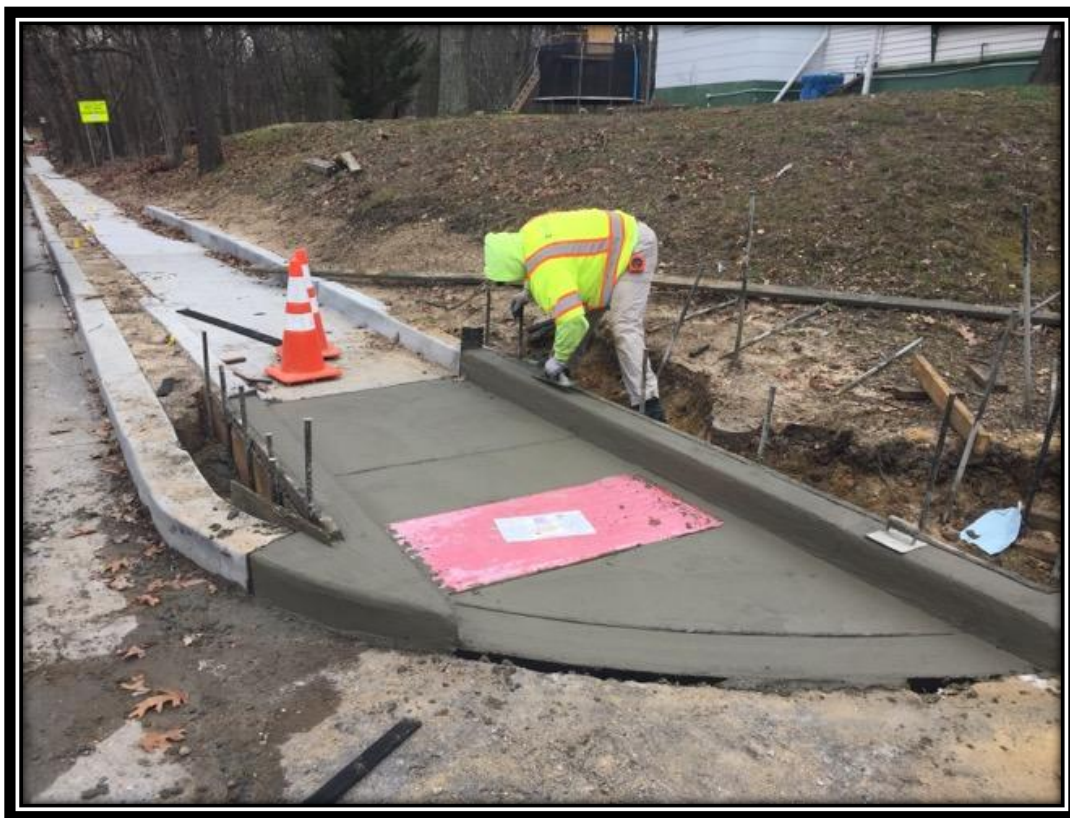
Figure: 1 – Installation of ADA ramp along the southbound lane at the intersection with Woodburn Avenue
