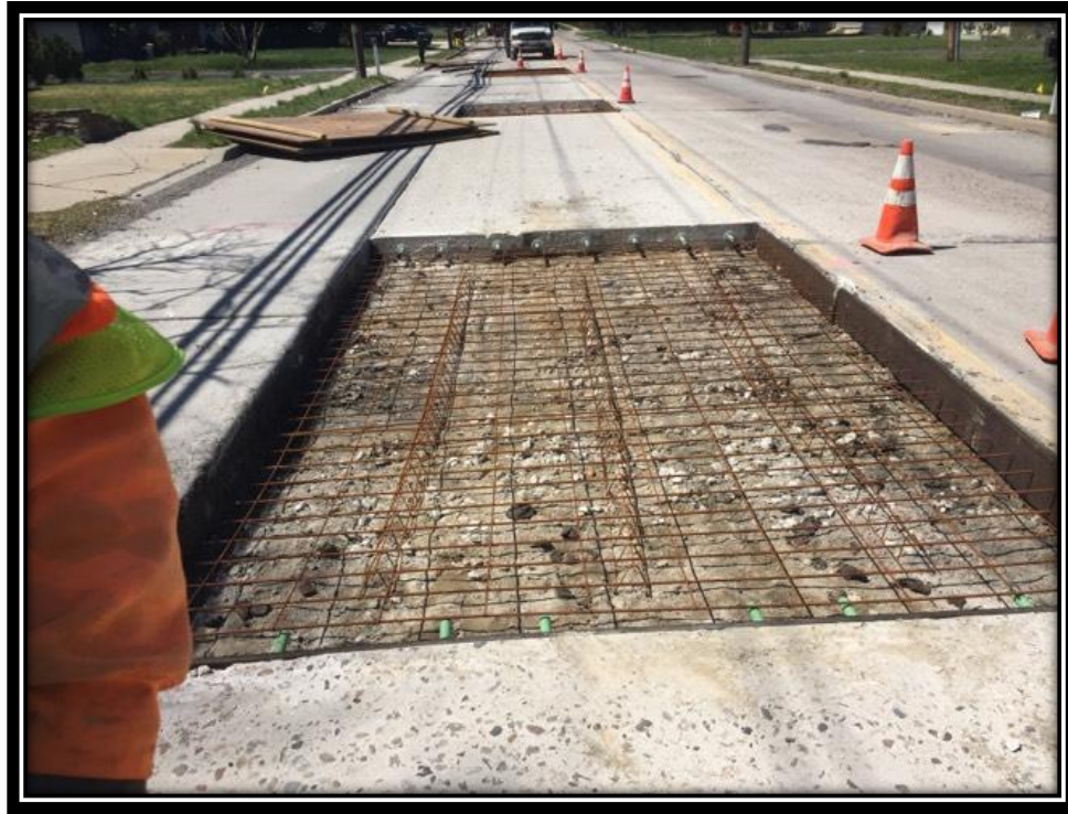
Figure: 2 – Full depth concrete slab repair along the northbound lane between Erial - New Brooklyn Road and Pleasantview Drive
