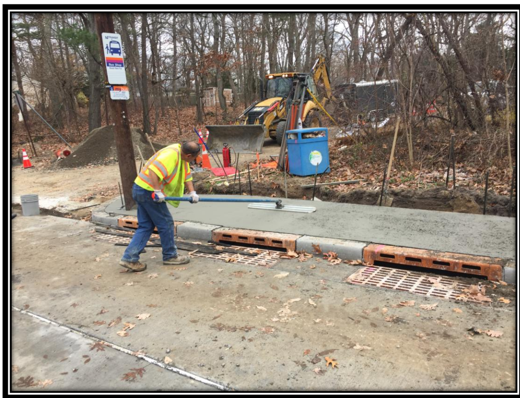
Figure: 1 – Installation of concrete sidewalk along the northbound lane at the intersection with Cloverdale Avenue
