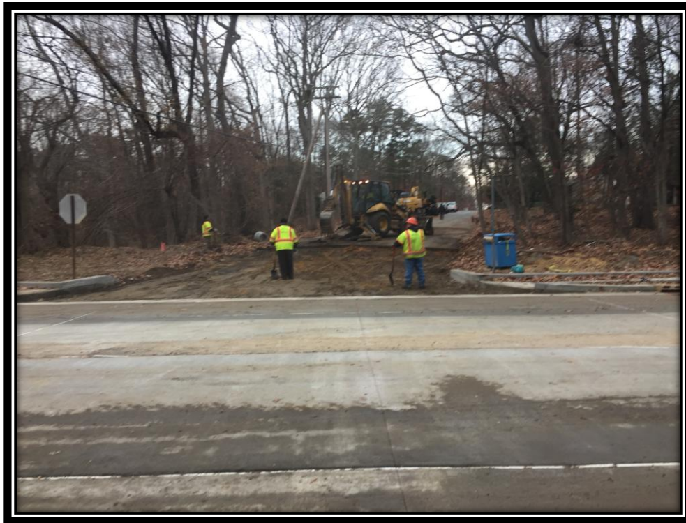
Figure: 2 – Excavation of the existing roadway at the intersection with Cloverdale Avenue
