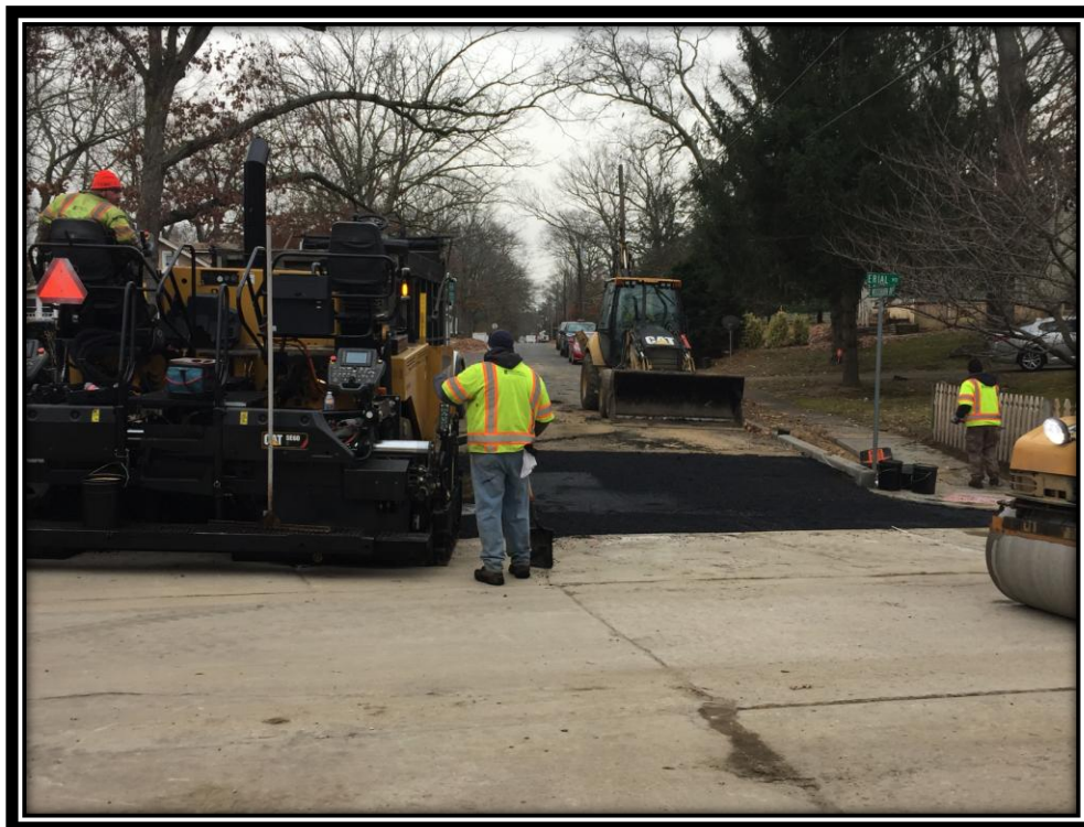
Figure: 3 – Installation of HMA 19M64 base course at the intersection with Woodburn Avenue
