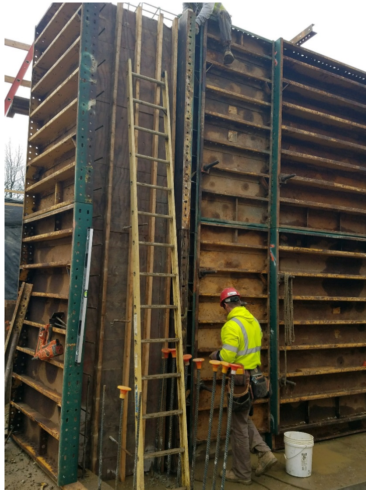
Figure 1 RE Pierson installing formwork at SE Abutment Wall
