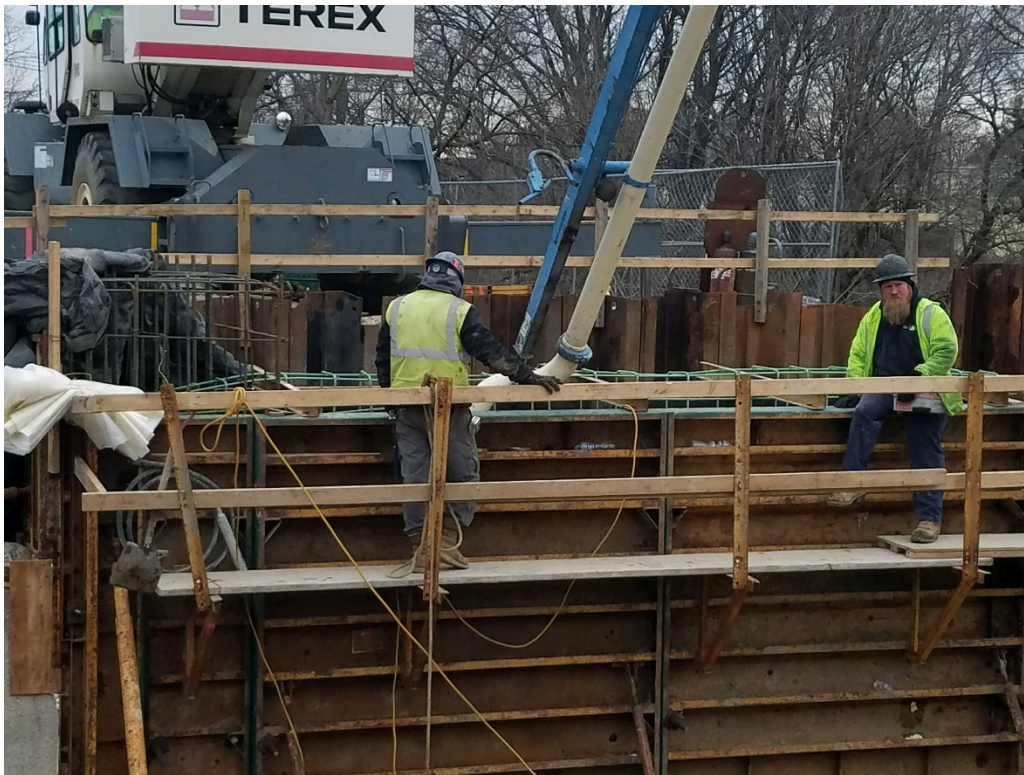
Figure 1 RE Pierson placing concrete at the northwest Abutment Wall
