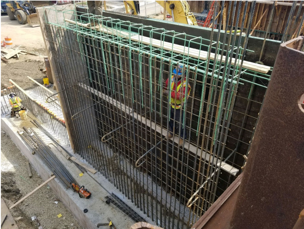
Figure 1 L&R Construction Installing Rebar on Abutment Wall.
