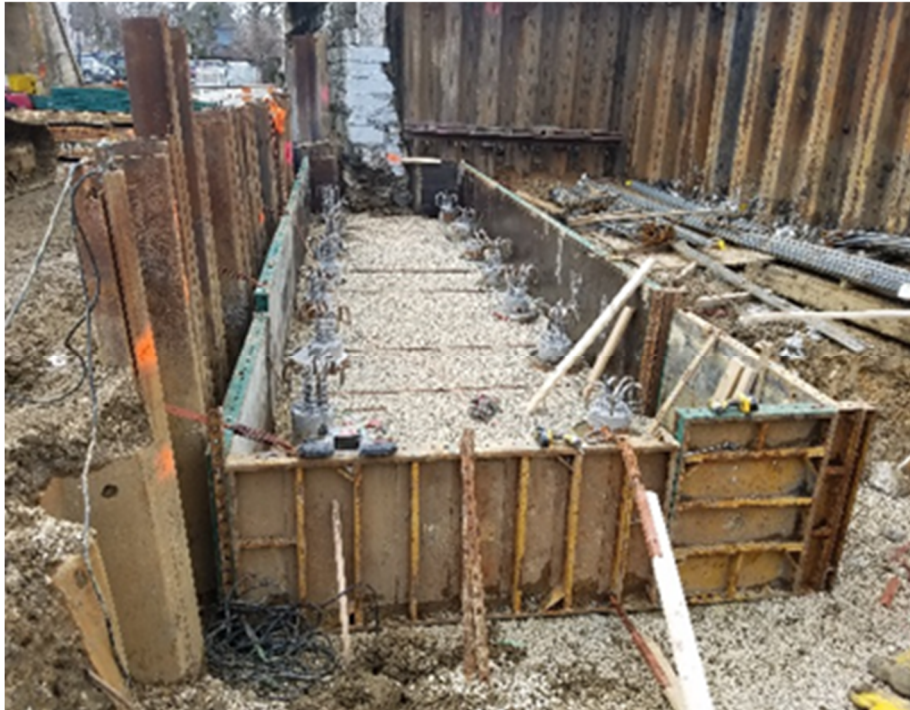
Figure 1 RE Pierson installing formwork at North Abutment Foundation
