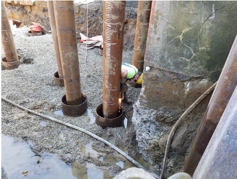
Figure 1 RE Pierson cutting off pipe pile at South Abutment
