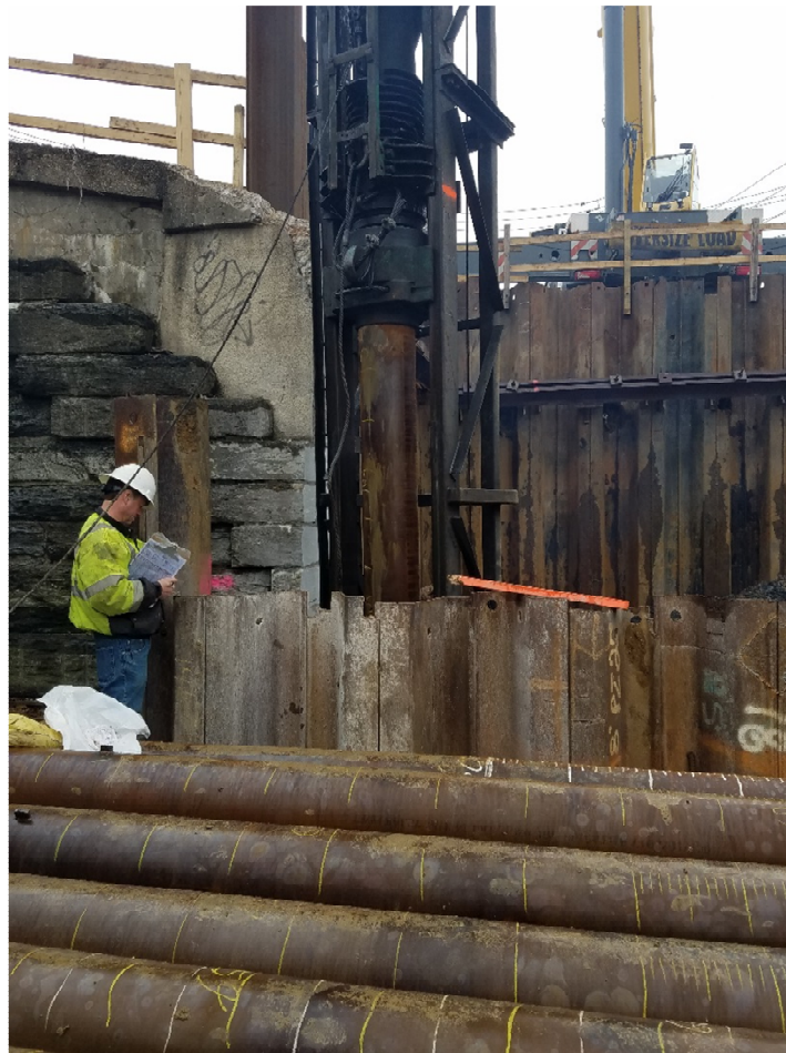
Figure 1 RE Pierson Driving Pipe Pile at North Abutment
