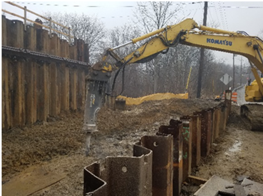
Figure 1 RE Pierson Demolishing North Abutment Footing
