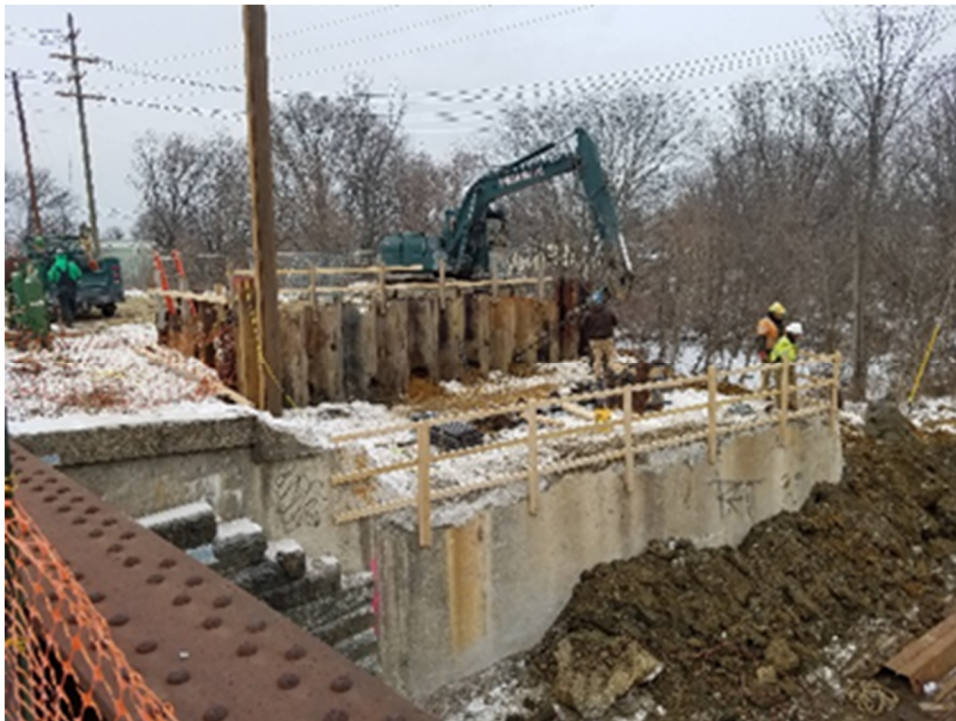
Figure 1 RE Pierson installing Safety Fence on North Abutment
