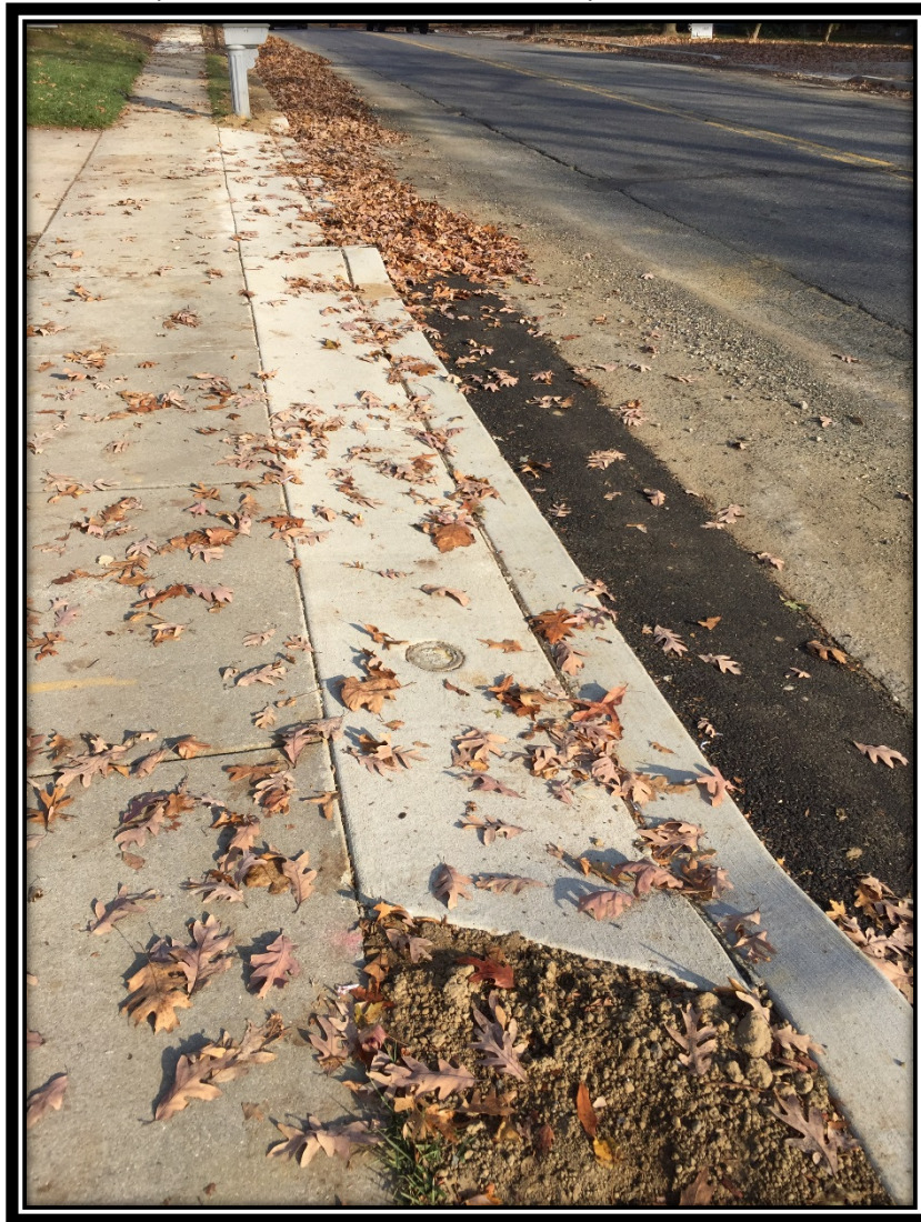
Figure 1 Concrete Aprons STA 120+50 Coles Road (LS)
