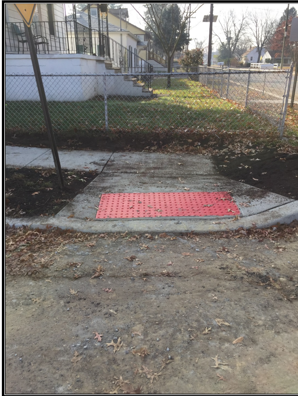
Figure 3 Handicap Ramp at Hassemer (East) STA 117+61 (RS)
