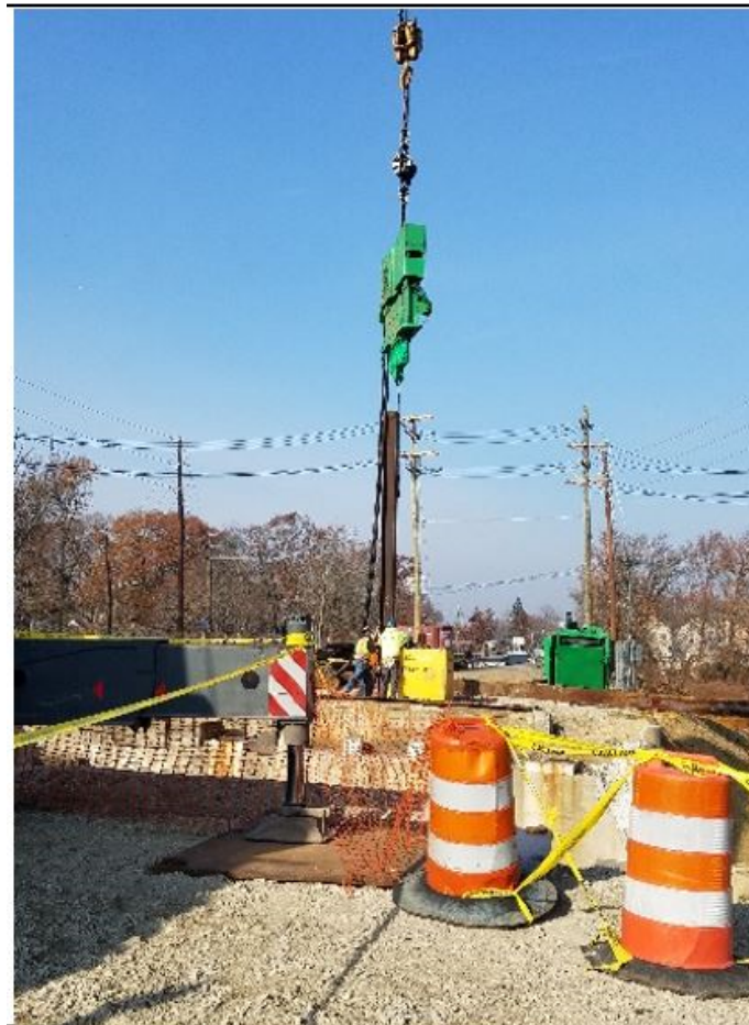
Figure 1 Driving H-Pile for Temporary Sheet Piling Template (North Side)
