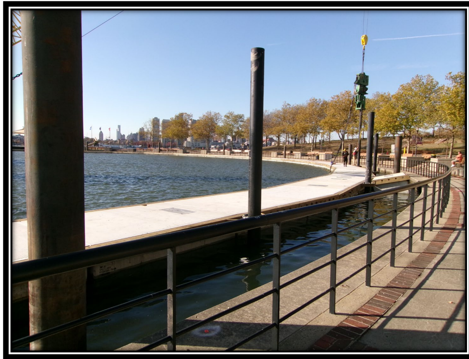
Figure: 2 – Driving of piles to secure newly installed circular concrete floating dock system at the southern end of the marina
