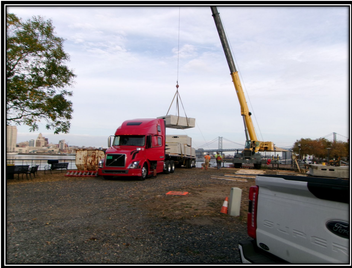
Figure: 1 – Unloading of newly delivered concrete floating dock sections
