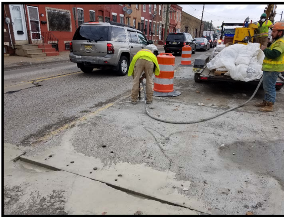
Pressure grouting of slab underside, joints and dowel pockets underway in Phase 1 work area.
