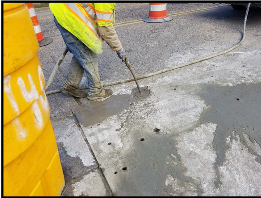
Pressure grouting of underslab in progress.
