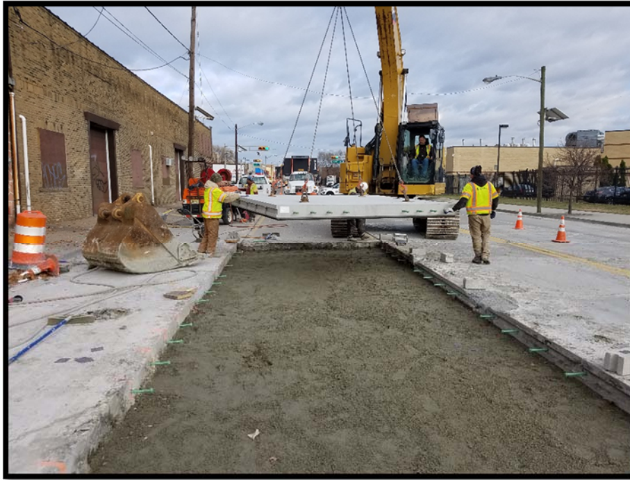
Installation of Phase 2 Slab in progress. Note work area encroaching on westbound travel lane resulting in police mandated lane closure and detour.
