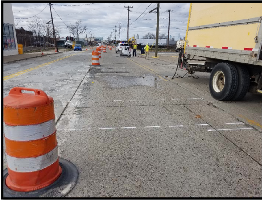
Phase 2 Temporary Traffic Striping and Drums installed. Traffic shifted to southernmost lanes and work zone in northernmost lanes. Sawcutting of Phase 2 slabs underway.
