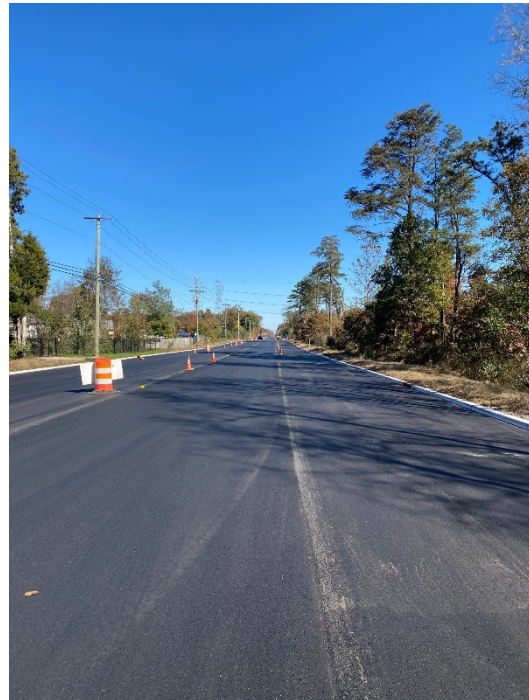
Figure 2: HMA Surface Course Placement
