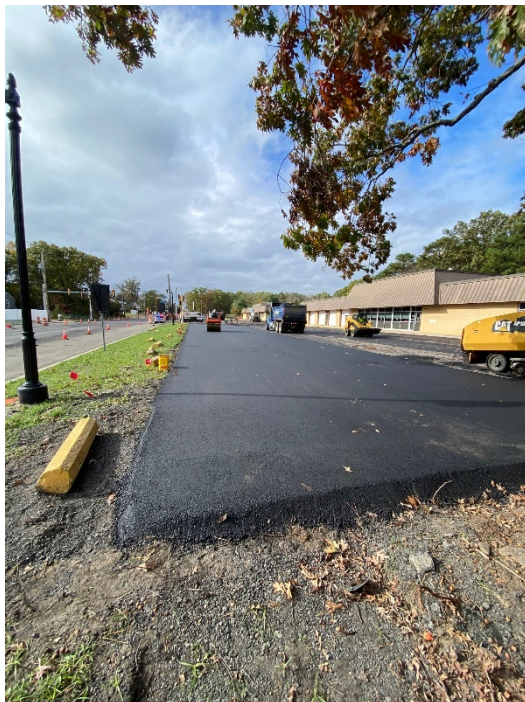
Figure 1: Camden School Driveway HMA Placement Figure 2: HMA Intermediate Course Placement
