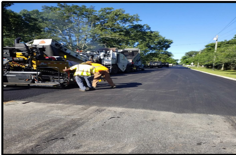
Photograph 3 – Surface Course Paving.
