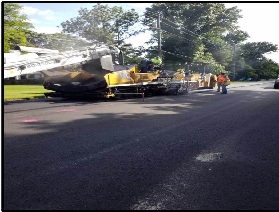
Photograph 1 – Paving Surface Course.
