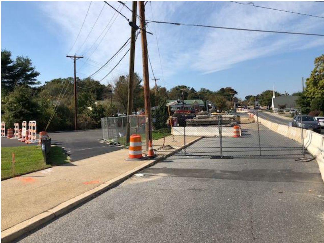
Contractor installed fence to keep pedestrians on the newly constructed walkway and out of the bridge demo work zone
