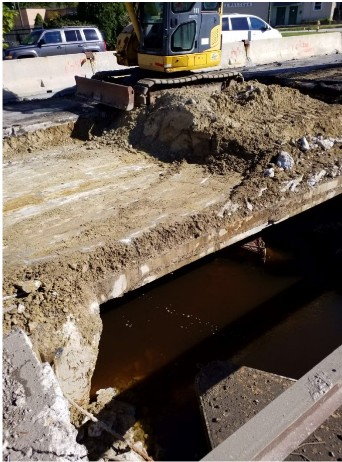
There was a layer of "dirt" between culvert box and concrete riding surface
