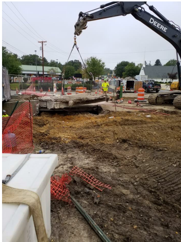
Removal of superstructure
