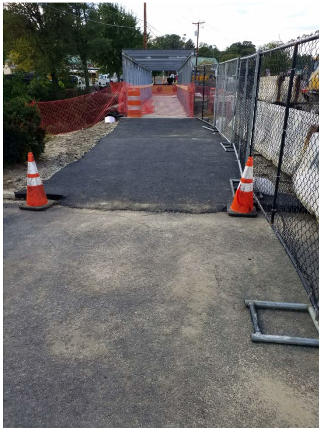
Asphalt sidewalk and fence installed. Temporary sidewalk is now open.
