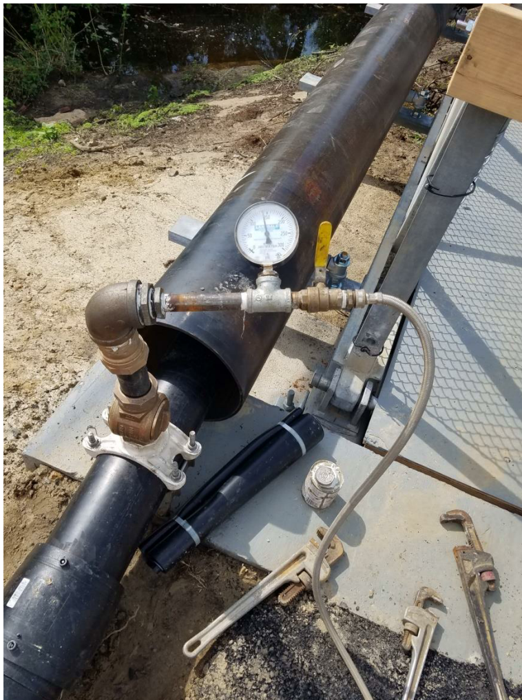
Water Main was pressure tested and choline tablets mixed in and tested.
