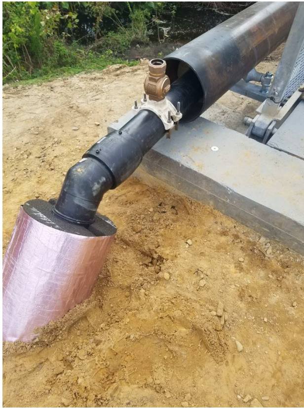
Water Main was insulated at each end and crossing the Pedestrian Bridge
