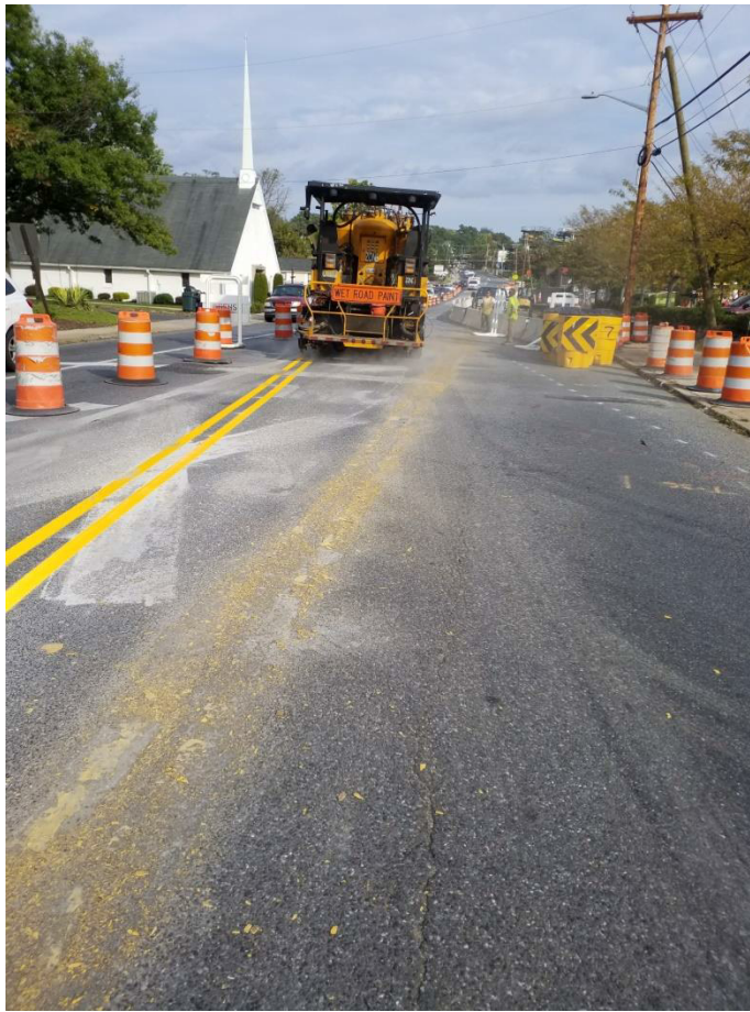
Old traffic stripes removed and new stripes installed for Stage 2 B of the project
