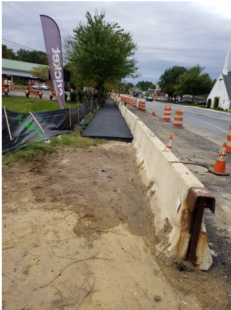
Temporary Sidewalk area was paved behind the newly placed Concrete Barrier Curb
