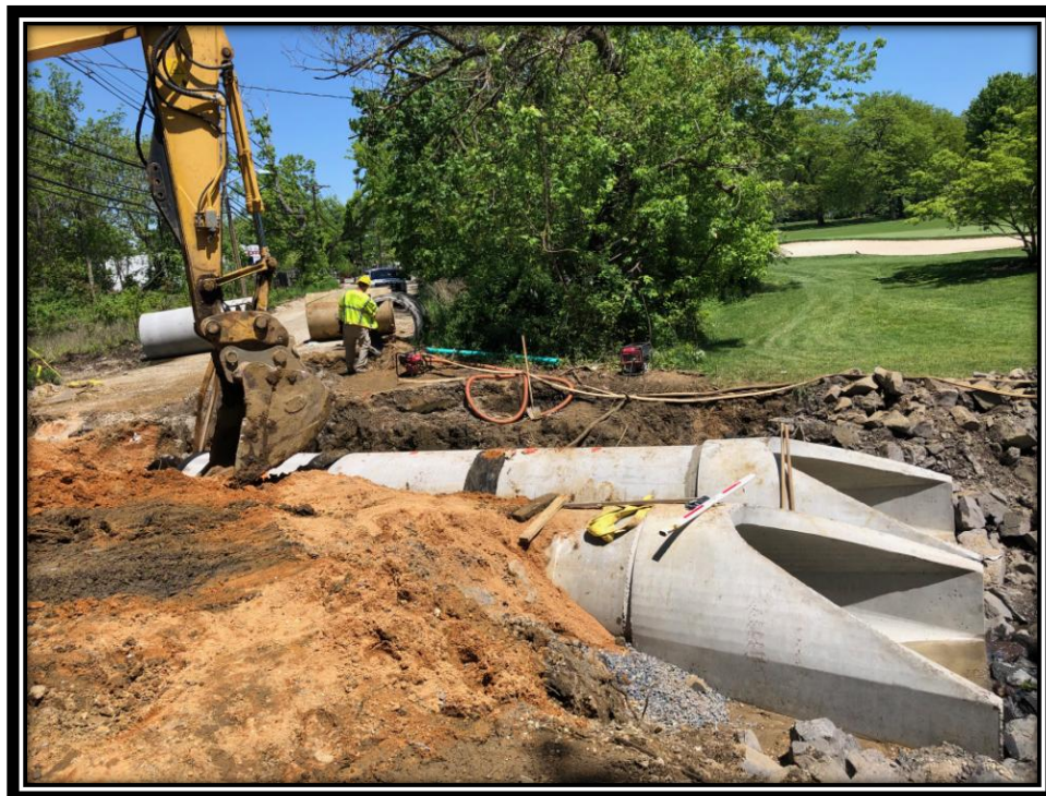
Figure: 3 – Installation of 48" RCP at the culvert replacement adjacent to the Merchantville Country Club
