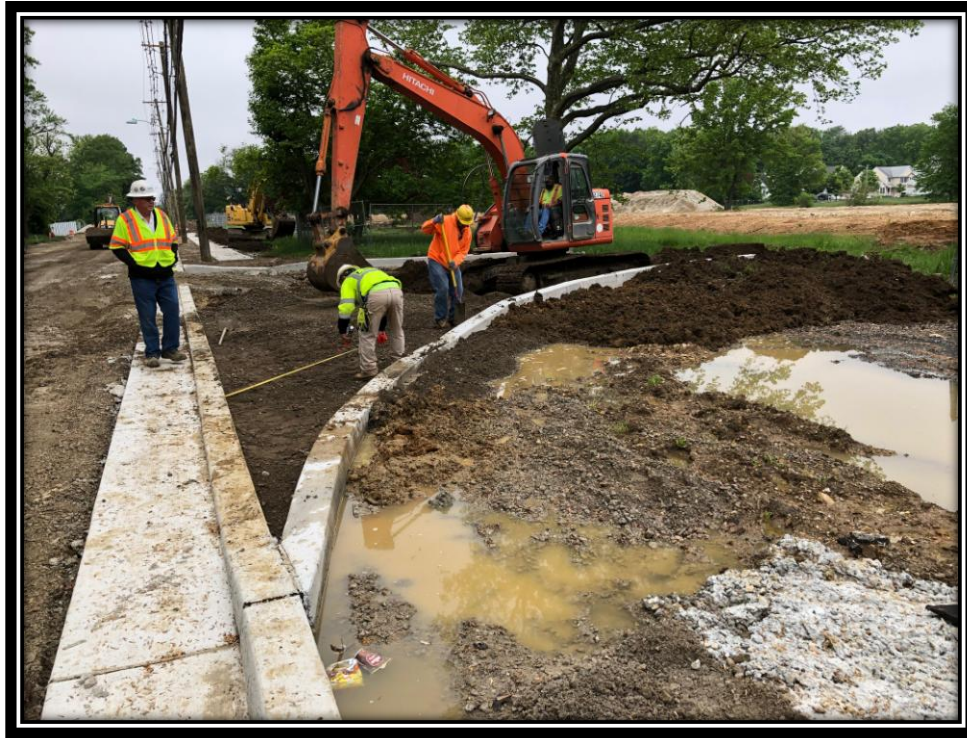
Figure: 2 – Installation of concrete curb & gutter and concrete vertical curb at future entrance to the proposed development along the westbound lane
