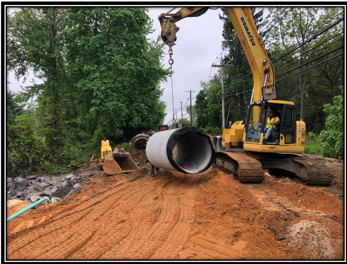
Figure: 1 – Installation of 48" RCP at the culvert replacement adjacent to the Merchantville Country Club
