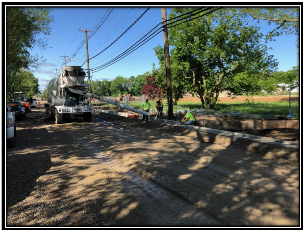
Figure: 3 – Installation of concrete curb and gutter along the westbound lane
