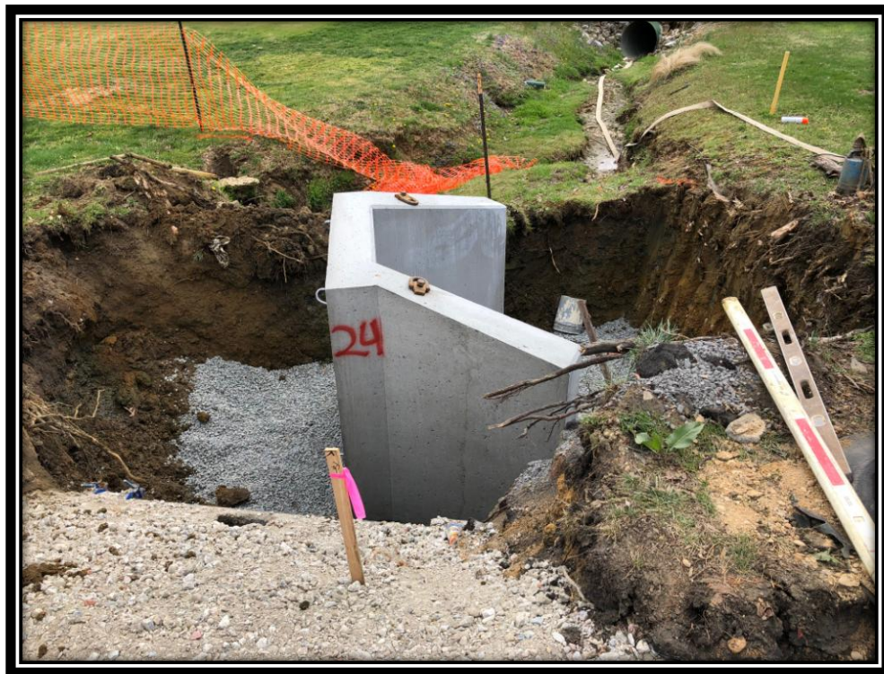
Figure: 3 – Installation of 24" concrete headwall along the northbound lane
