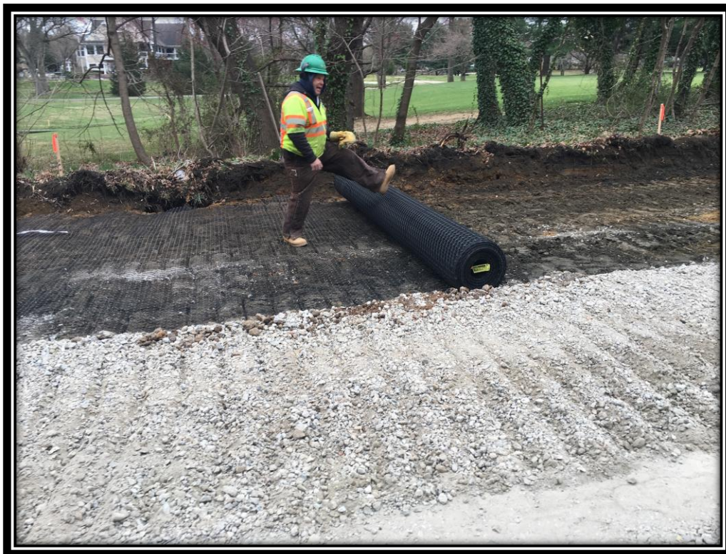
Figure: 3 – Installation of 6" thick dense graded aggregate base course in the southbound lane and pavement reinforcing geogrid along the northbound lane
