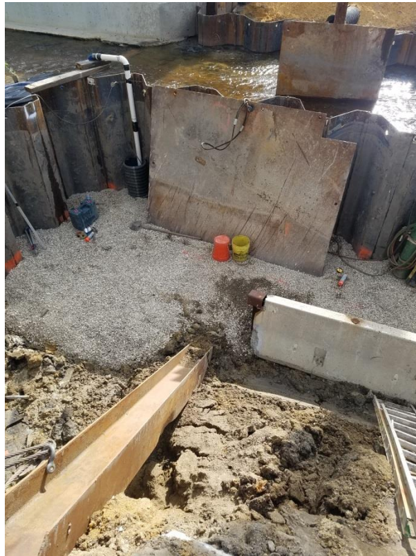
Stone bed installed for footing
