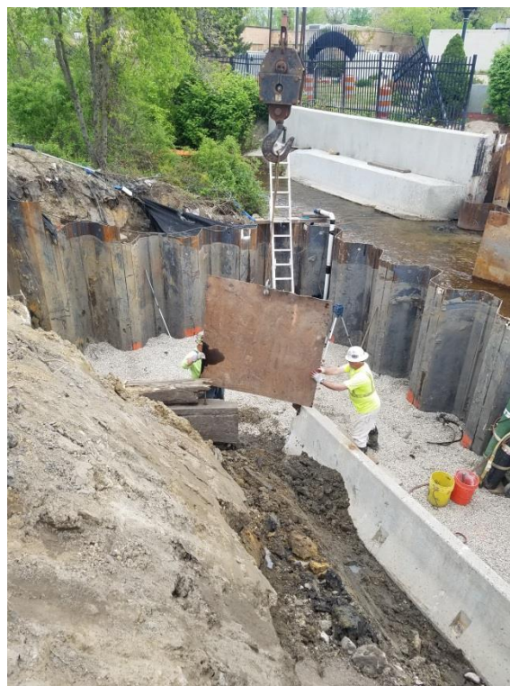
Shoring installed for workers safety
