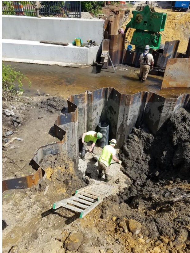
Sump pit installed for dewatering operation
