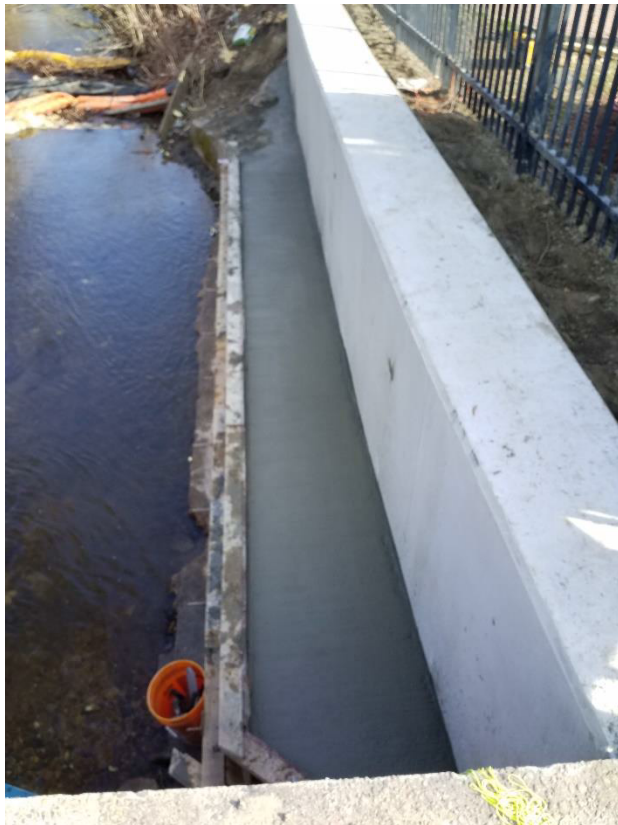
After lower wall was poured to replace in kind of the existing condition
