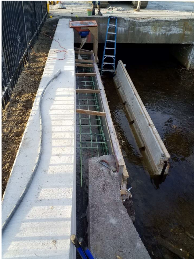
Re-steel and forms in place for the lower seat wall
