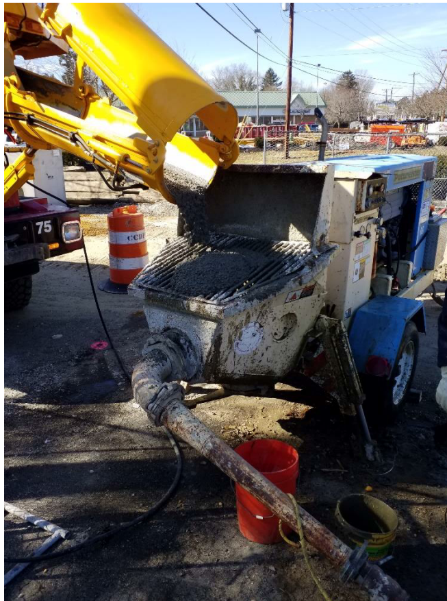
Contractor using a portable concrete pump to pour concrete between culvert and steel sheets
