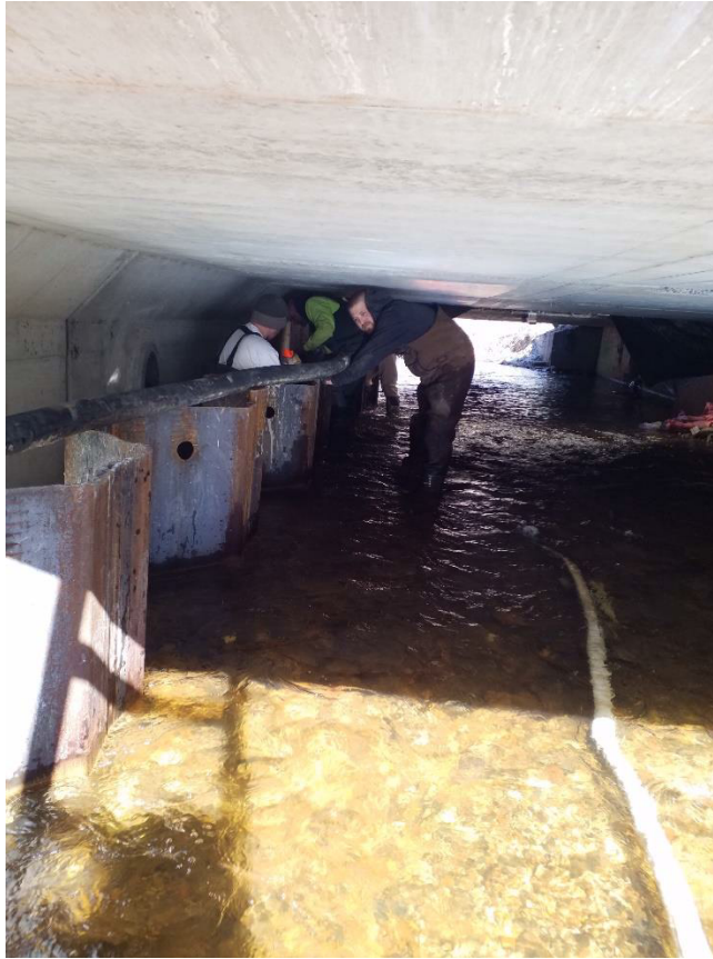
Concrete was both under the culvert and in front of the 2-wingwalls
