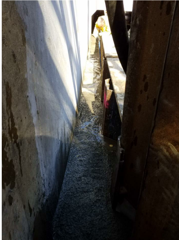
Concrete being place to a known grade behind steel sheets
