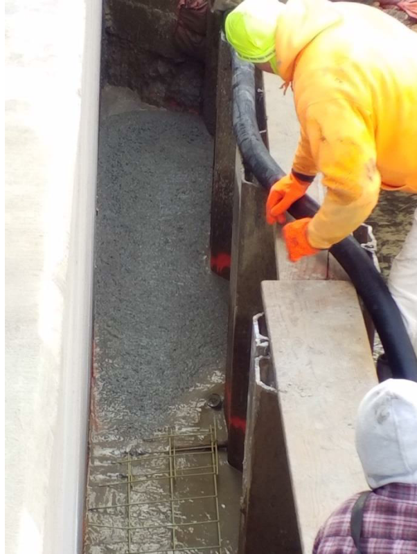
Pumping concrete where wire mess was installed
