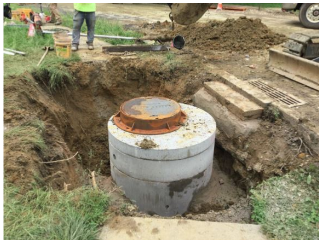
Figure 1: Doghouse manhole installed
