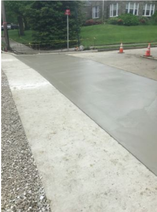
Figure 2: Concrete swale at King Ave
