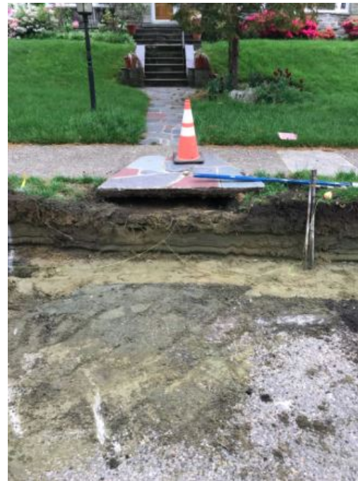
Figure 3: Demolition of Flag Stone, Plan for Exposed Aggregate Sidewalk Replacement
