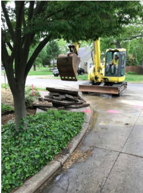
Figure 2: Demolition of Existing Curb Ramp
