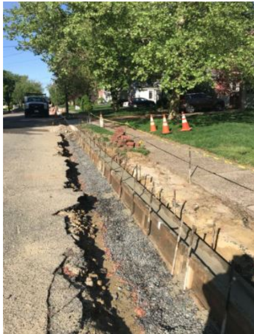
Figure 1: Concrete Curb Poured in Forms
