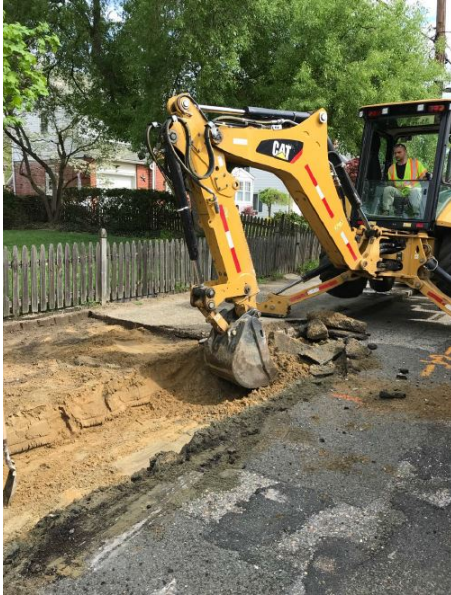
Figure 2: Demolition of Concrete Sidewalk
