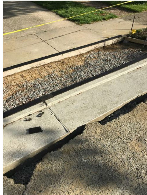
Figure 3: Installation of Concrete Gutter and Driveway
