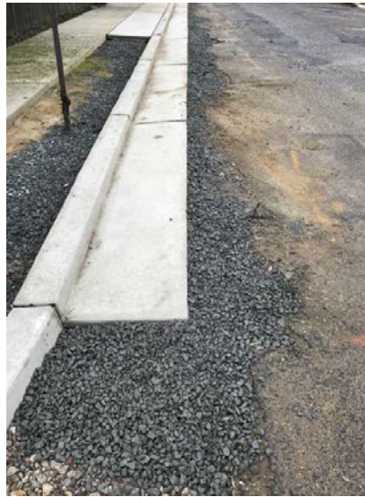
Figure 1: Concrete Curb and Gutter Installed
