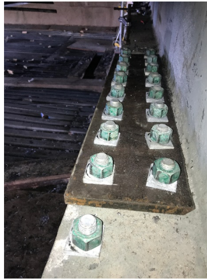
Figure 1: Cuthbert Blvd. Bridge – Steel Installation
