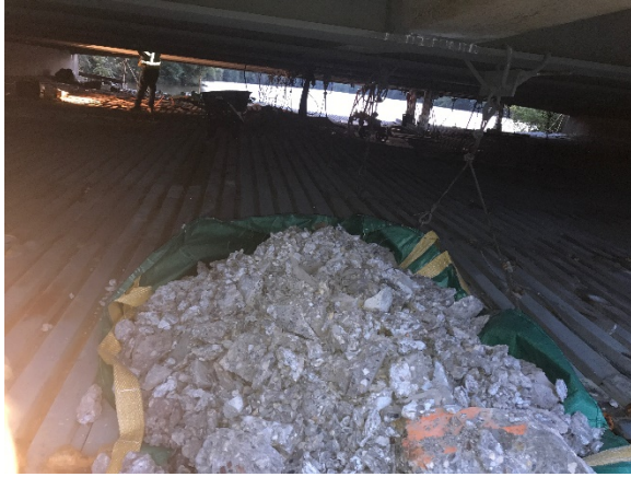
Figure 2: Cuthbert Blvd. Bridge – Diaphragm Demolition
