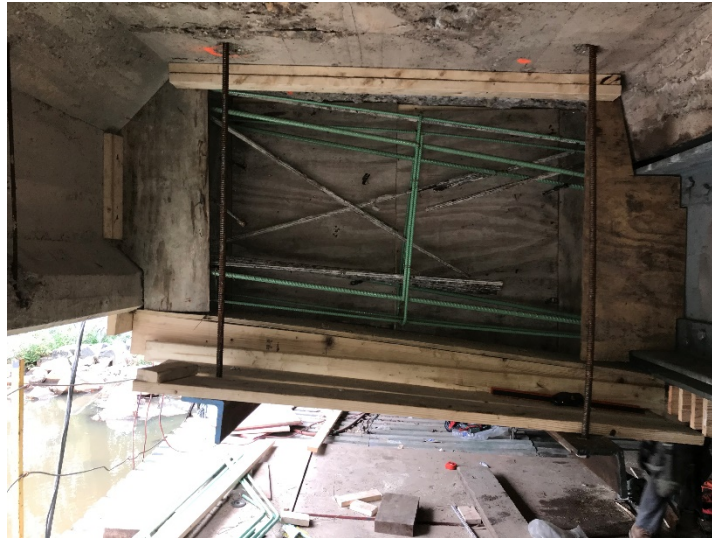
Figure 1: Grove St. Bridge – Rebar and Formwork between G9 and G8
