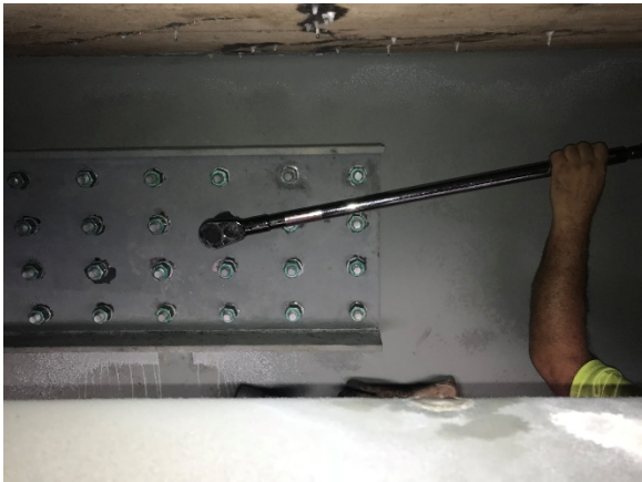
Figure 3: Grove St. Bridge Bolt Testing
