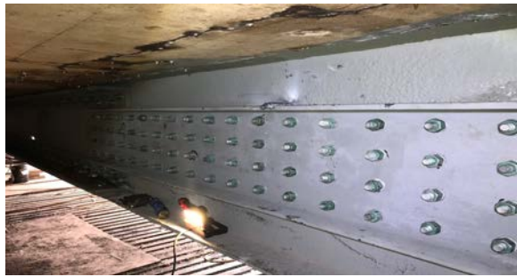
Figure 2: Grove St. Bridge Installation of Structural Steel Channel Beam G-8
