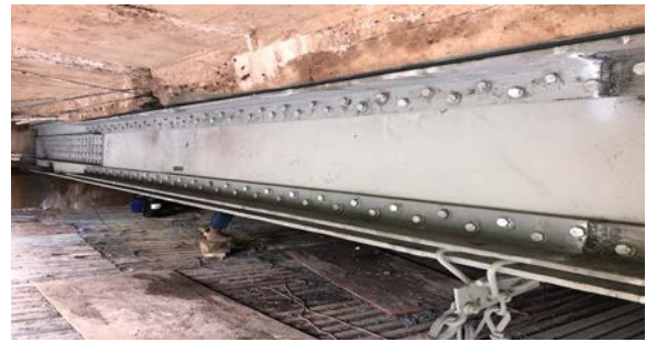
Figure 3: Grove St. Bridge Installation of Structural Steel Channel Beam G-9
