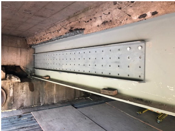
Figure 2: Grove St. Bridge Installation of Structural Steel Channel Beam G-9
