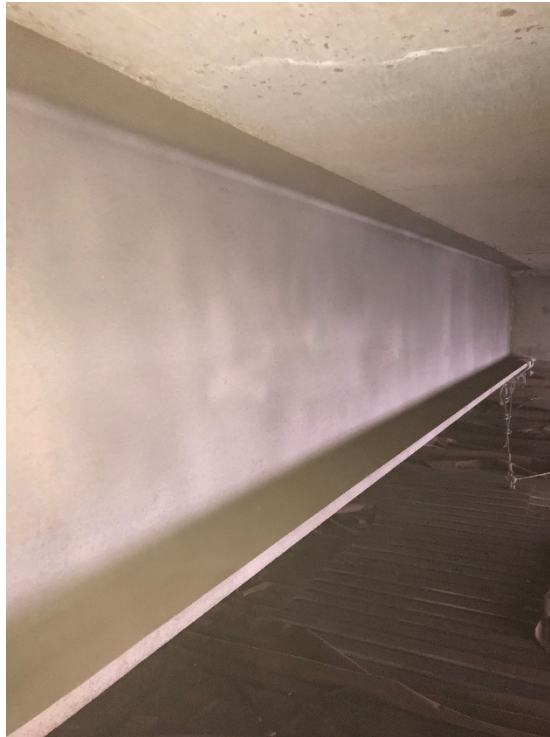
Figure 2: Cuthbert Blvd. Bridge Prime Coat
