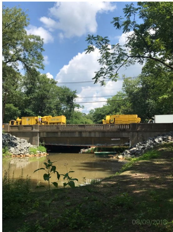
Figure 1: Grove St. Bridge Near-White Blast & Paint
