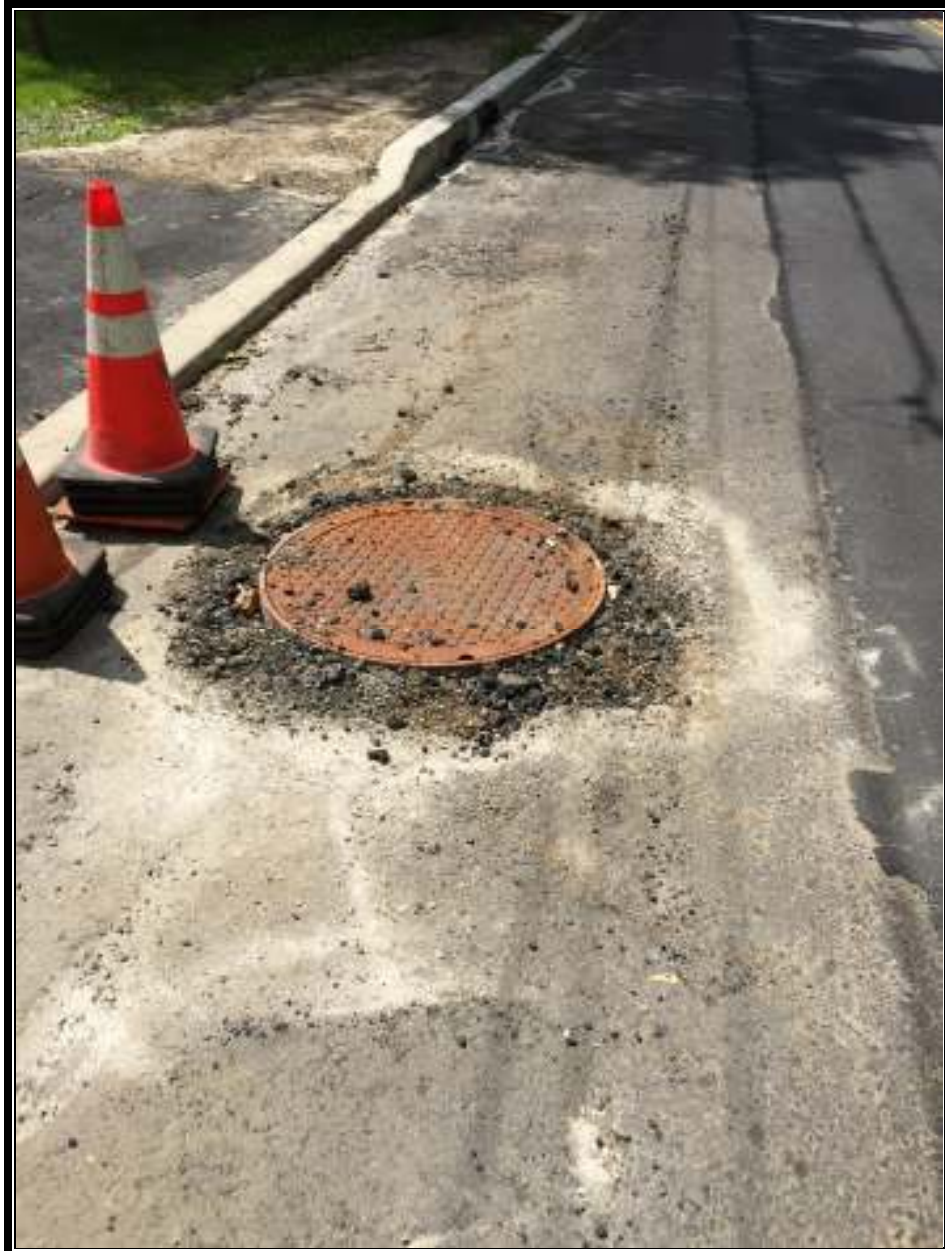
Figure 2 New Reset Manhole Casting
