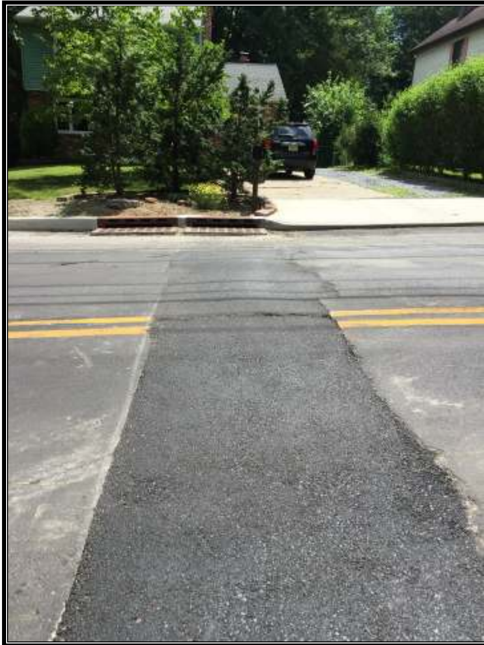
Figure 3 Concrete Joint Repair
