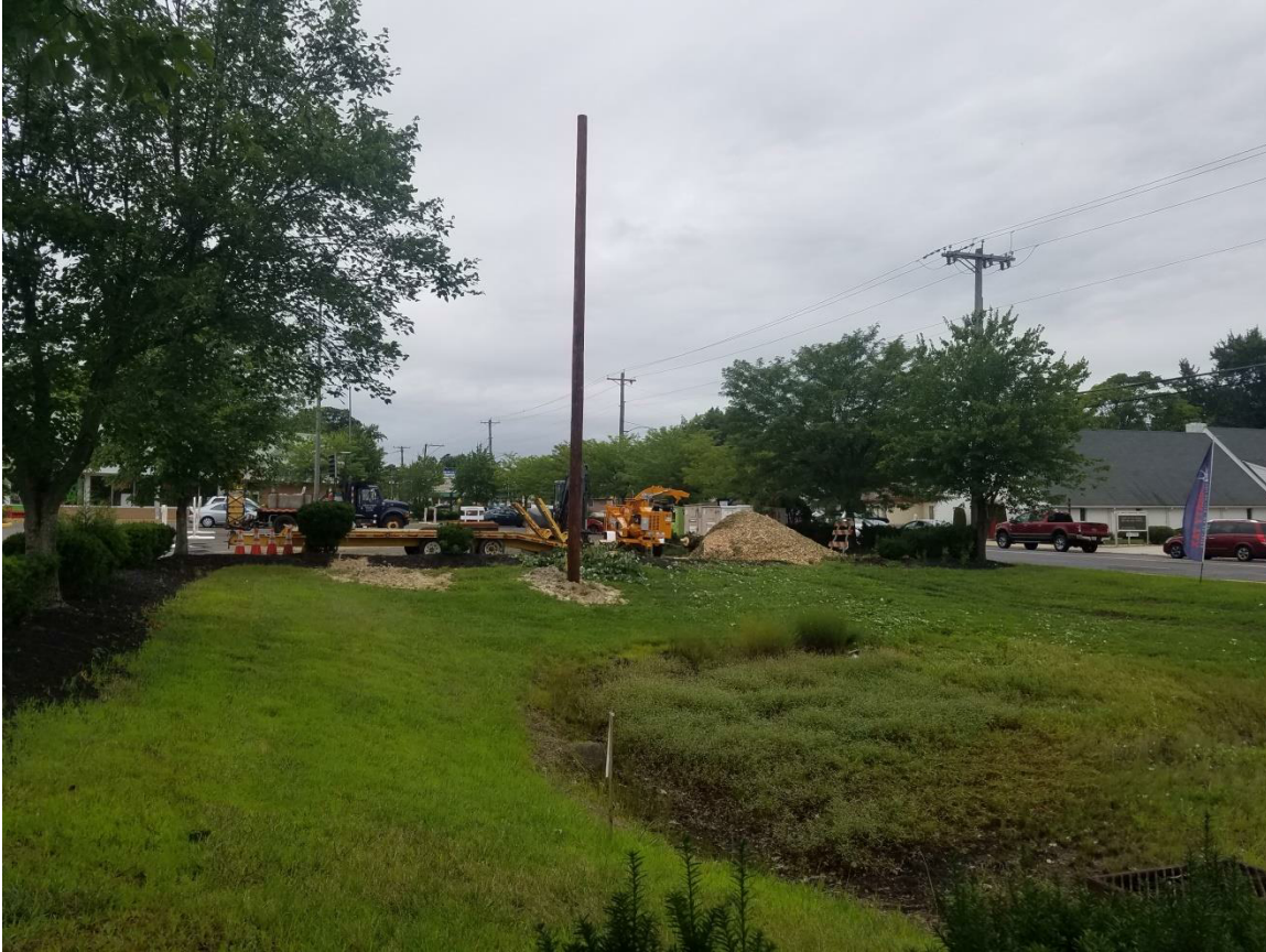
Temporary Pole set for Aerial lines to be relocated.
