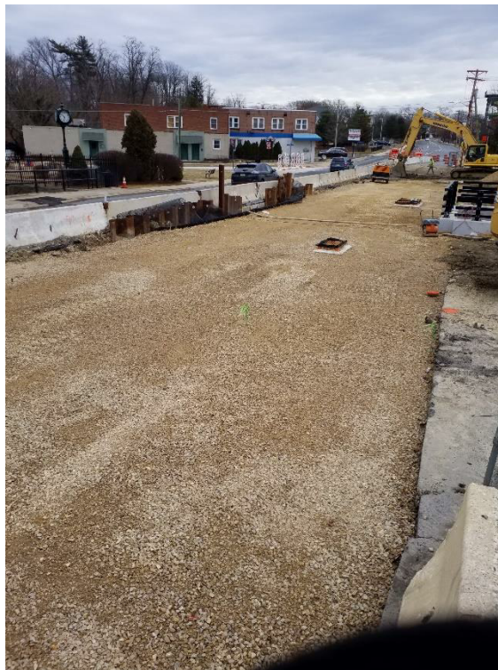
Again looking east at the DGA that was placed in roadway section for Stage 2B
