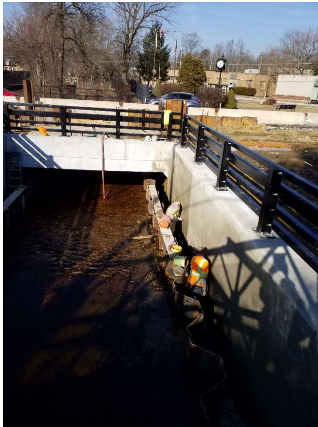
Contractor rubbing wingwall
