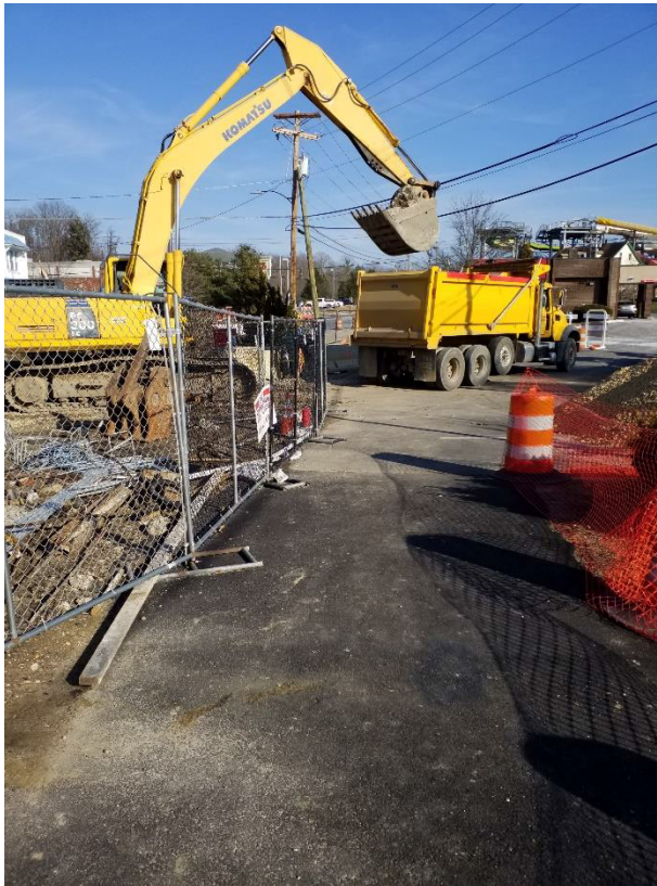
Contractor removed the existing concrete roadway to enable new roadway to be build to plan grades
