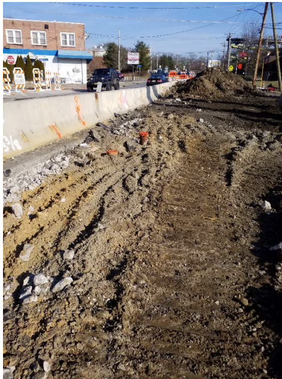
Section of boxed out roadway once concrete was removed
