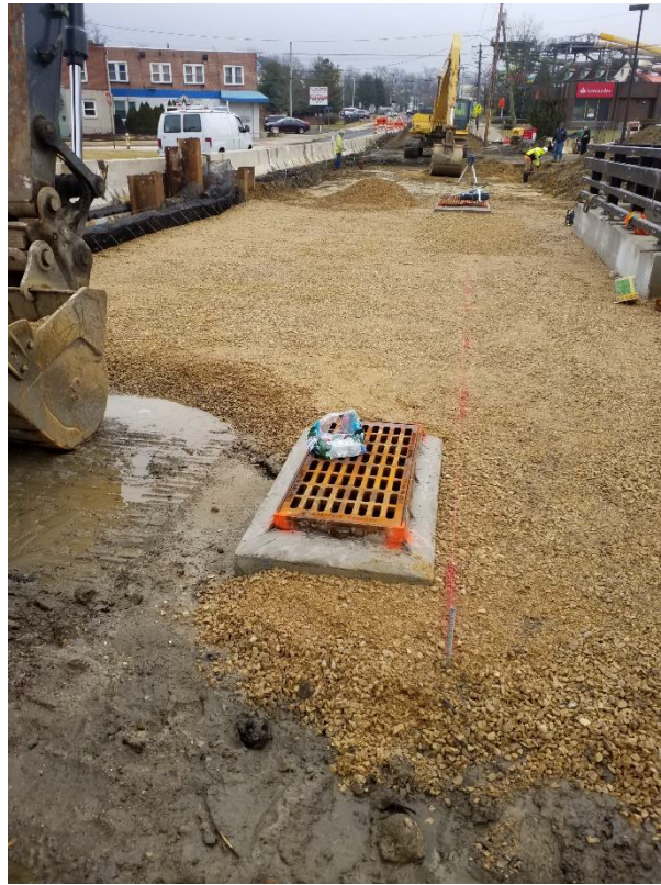
Placement of DGA over culvert section and in roadway
